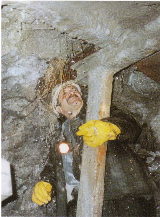
Biggest task was to support the ground over the cutterhead.
