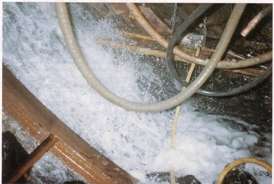
Around 5,000 l/min of water was encountered at the site of the roof fall.
