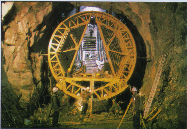
Full round conical shaped form assembled for the James Bay hydro project in Quebec. EFCO supplied 5200ft 2 of special all steel forms to Spino Construction Co to form the 6300ft long penstock tunnels. These forms were used to cast the 80ft long interior elbow. Because of its conical shape, EFCO manufactured 17 trussed sections located on 4ft centres with increasing diameter to adjust from the bottom 22ft diameter to the top 26ft diameter.
